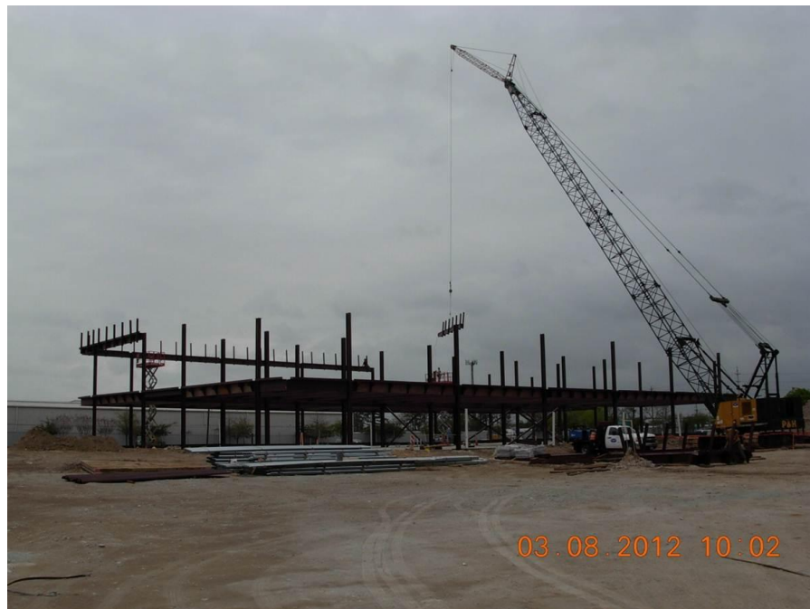
Figure 3: Structural Steel Frame - Image Provided by Tutor Perini
