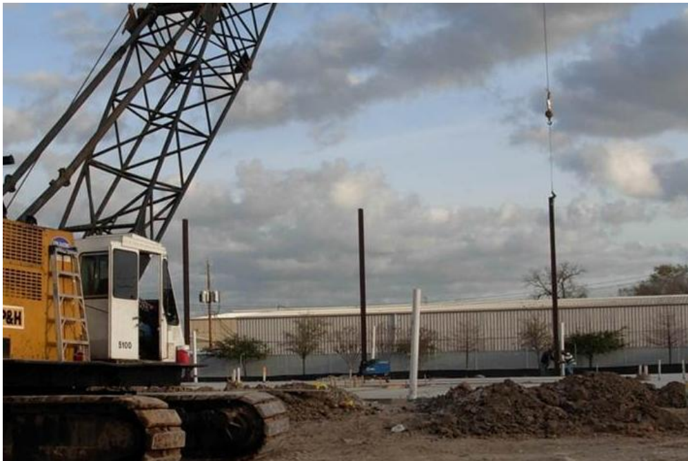
Figure 2: Column Erection - Image Provided by Tutor Perini
